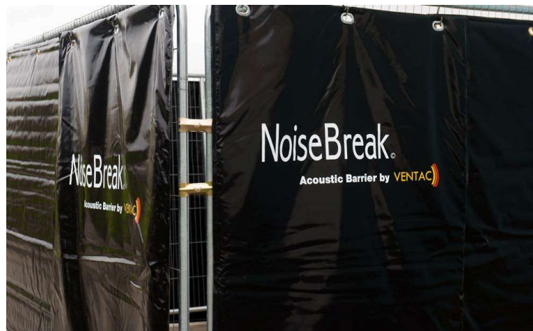
Figure 10-10 Temporary Construction Noise Barrier © Ventac
